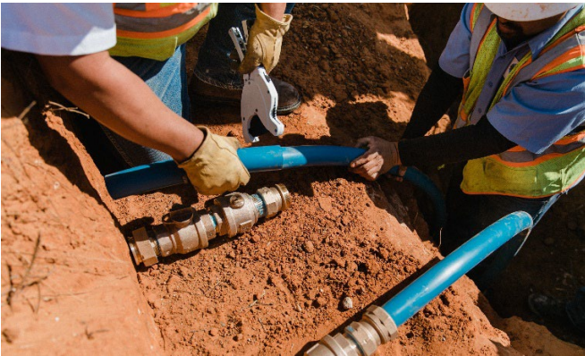
The updated AWWA C904-22 can help installers meet the rapidly growing need to replace lead pipes with PEX. Photo courtesy of PPI-member company REHAU.
